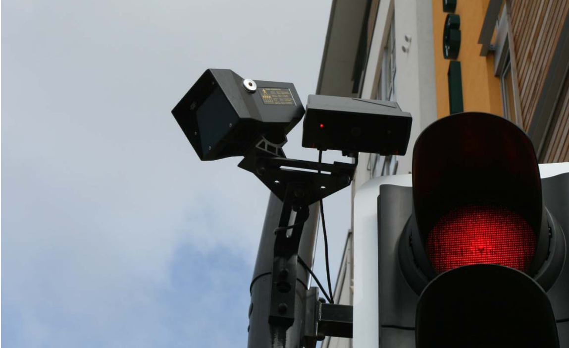
Figure 2. Automated Pedestrian Sensors are Used to Adapt Signal Timing for Pedestrians (Bristol, United Kingdom)
